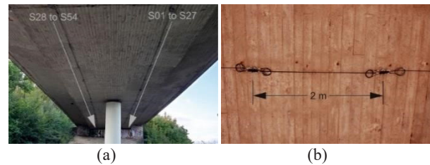
Figure 3 – Overview of the bridge and the monitoring system: (a) Sensor distribution; (b) An LGFBG sensor with a 2.05 m gauge.
